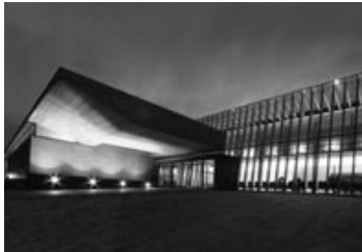
LG Medal Winner Prince George Airport Expansion, Prince George BC Firm: mcfarlaneGreen Architecture + Design Inc. Lead Design Architects: Michael Green MAIBC, Steve McFarlane MAIBC, Vicki Brown MArch.
