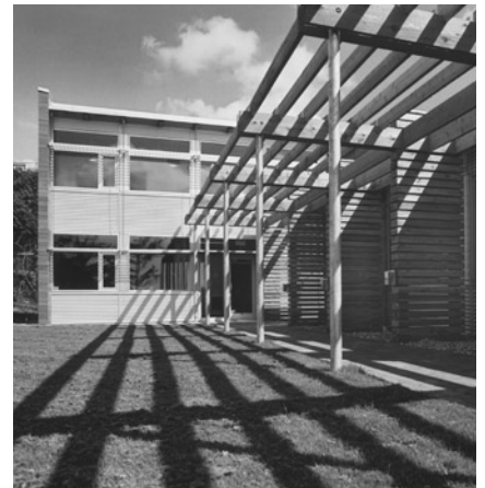
White Rock Operations Building, White Rock, BC
