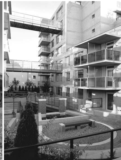
LORE KRILL HOUSING CO-OP + City of Vancouver Parkade Vancouver, BC
